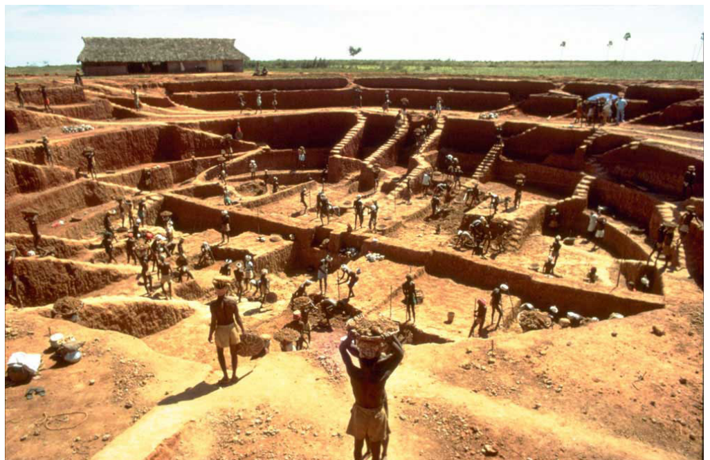
Excavating the foundation crater for Matrimandir in 1971
