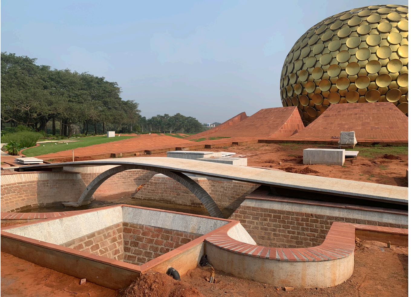
The newly completed arching bridge in the Garden of Utility
